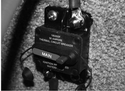
The power to the dash circuit is protected by a circuit breaker that is located in the observer seat storage area near the battery.
